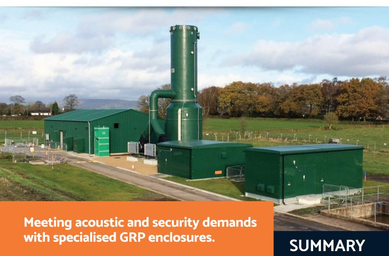
This project required a specialised solution to meet the client's specific acoustic and security needs, particularly in a densely populated area where noise prevention is crucial. To address these requirements, an SR4-rated GRP enclosure with an impressive acoustic rating of up to 30dB was selected. This level of noise reduction is highly sought after in urban environments where noise control is a priority for minimising disruption.
