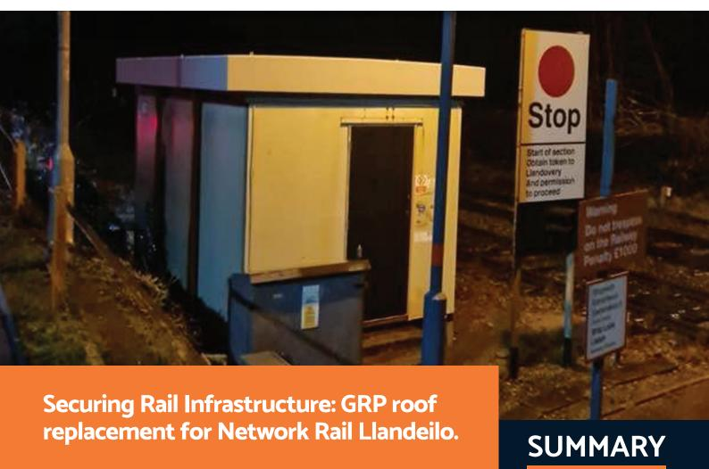
Network Rail commissioned a GRP roof replacement for an existing relay room at their Llandeilo site in Wales. With budget constraints preventing the full replacement of aging kiosks and buildings, a cost-effective yet high-performance solution was required to ensure continued protection of critical railway infrastructure from the elements.
